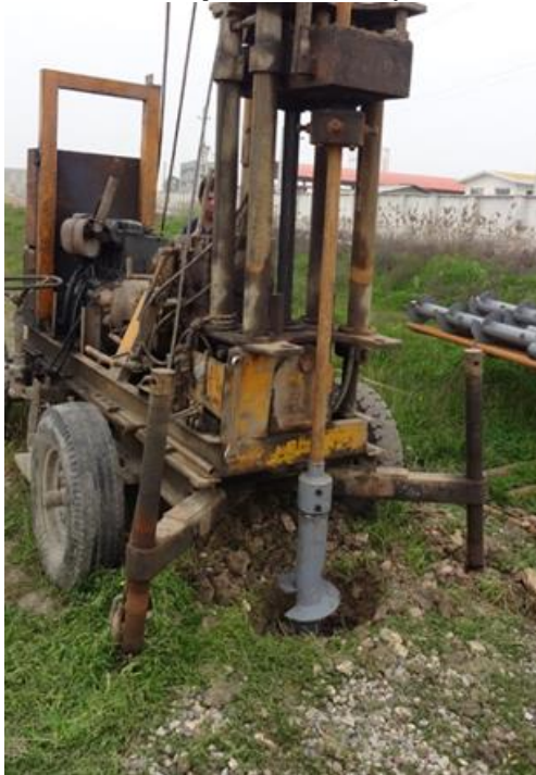
Figure 5. Helical pile installation equipment
