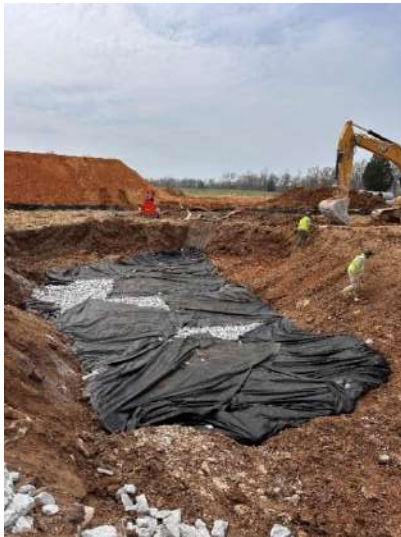
Figure 1. a to e) Sinkhole Remediation via Inverted Rock Filter
