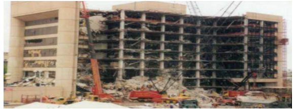
Fig.1. Progressive collapse in Alfred P Murrah
