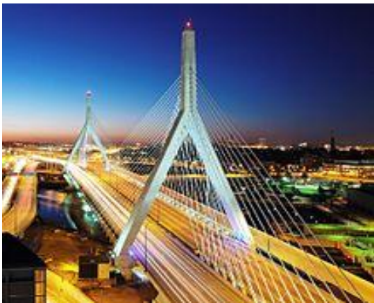
Fig. 2. Cable stayed bridge A shape tower
