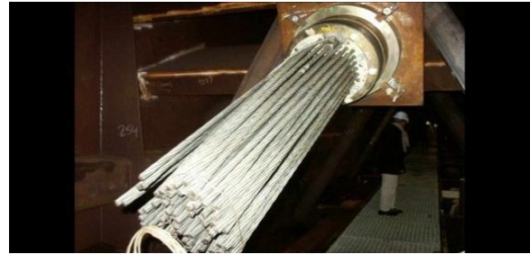
Fig. 1. Spiral strings coated by a shield
