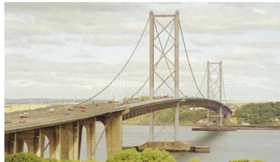
Fig. 3. Suspension bridges with parabolic cables
