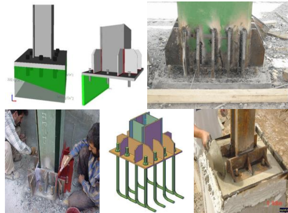
Fig.11 column plates installation
