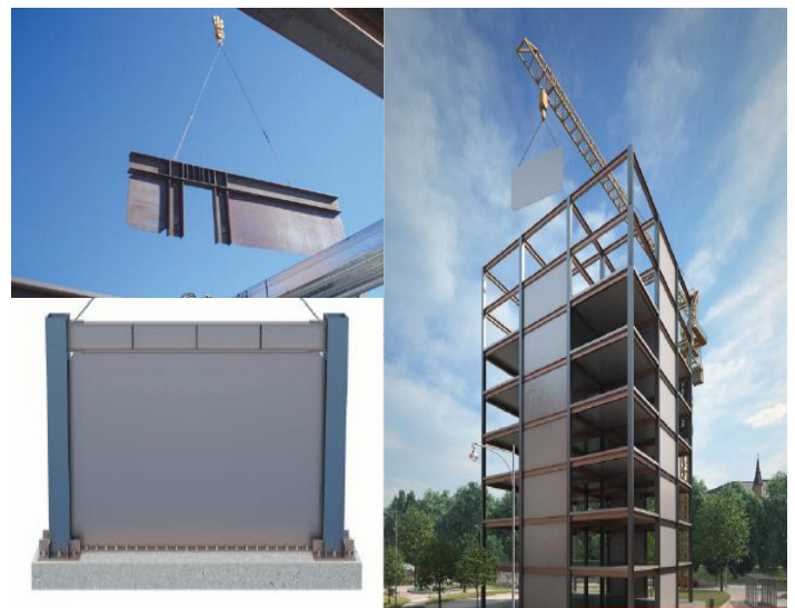
Fig.12 Carriage and installation of steel shear walls
