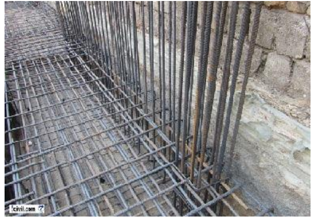
Fig.7 Shear wall's starter bars placing
