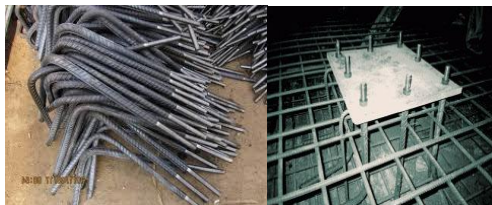
Fig.10 shear wall's Anker bolts
