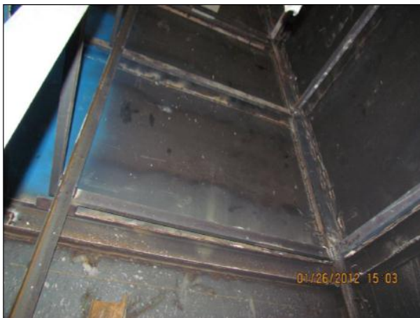
Fig.14 Steel shear walls installed by welding
