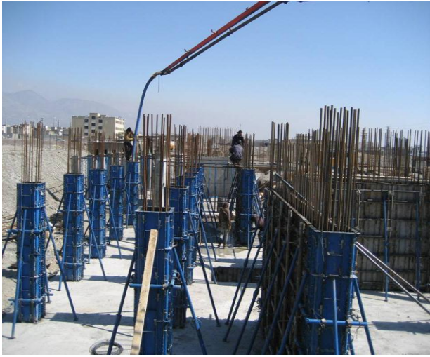
Fig.9 formworks installation and concrete pouring
