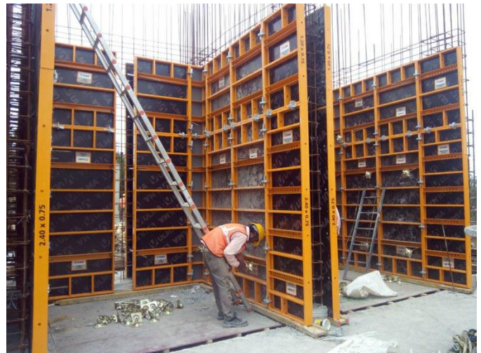
Fig.8 formworks installation
