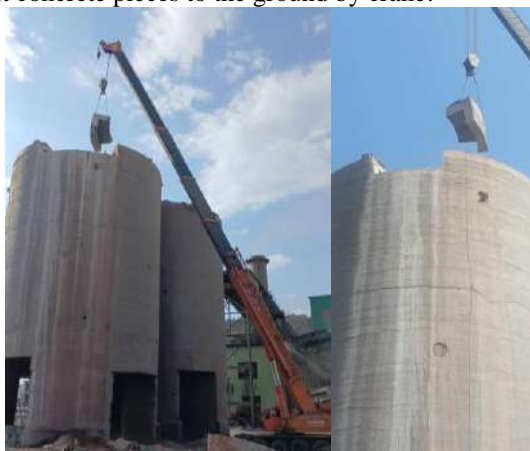
Figure 11. Transferring the cut concrete piece to the ground by crane
