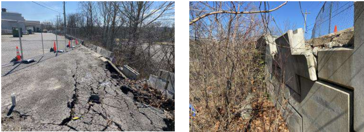
Figures 2a and 2b) The current state of the failed retaining wall
