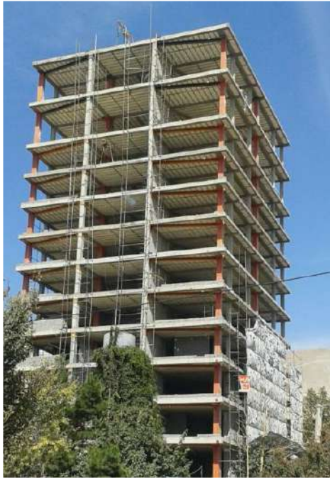
Fig. 7. The building retrofitted by steel jacking
