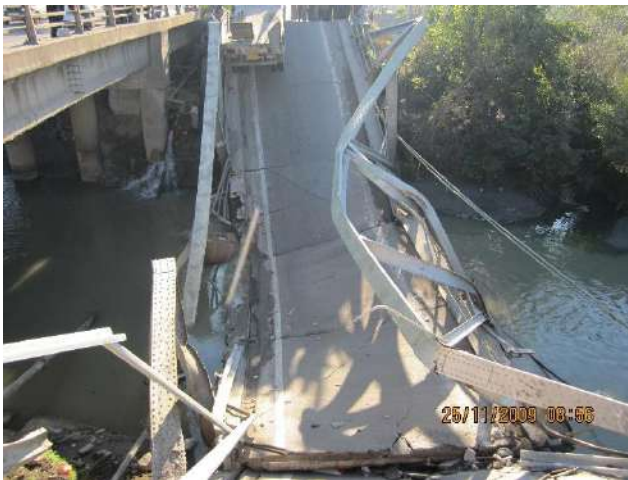
Fig. 2. the collapse of Sardabroud bridge due to heavy load collision with a key element of the structure
