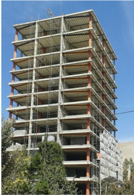
Fig. 7. The building retrofitted by steel jacking
