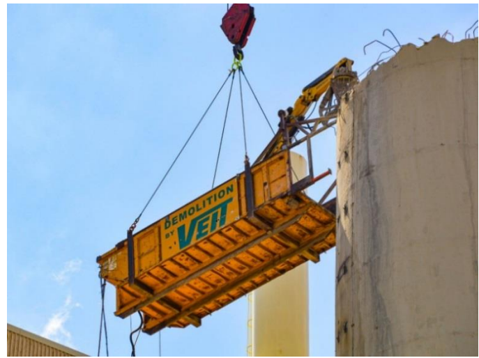
Figure 4. Transferring the shovel on a metal platform by a dry boom crane at a height for demolition by a hydraulic jaw (scissors) or a pickaxe in stages from top to bottom
