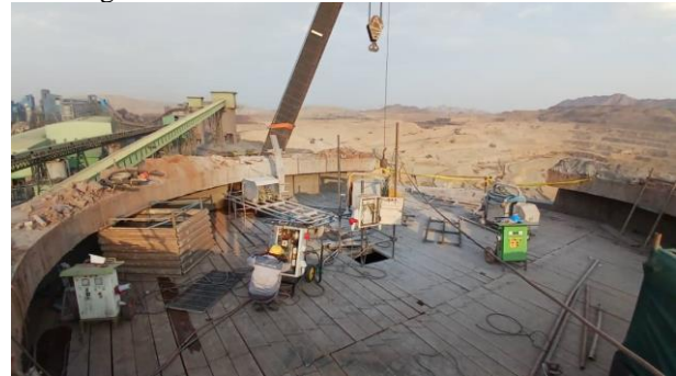
Figure 9. Simultaneous creation of three work fronts in the concrete wire cutting demolition method (simultaneous use of two horizontal and vertical cutting machines along with a concrete cutter)
