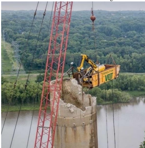
Figure 4. Transferring the shovel on a metal platform by a dry boom crane at a height for demolition by a hydraulic jaw (scissors) or a pickaxe in stages from top to bottom
