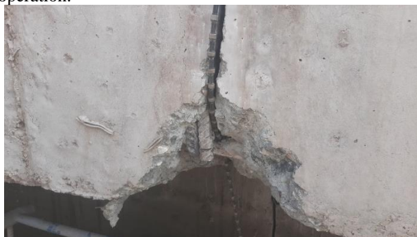
Figure 10. Tearing of cutting wire at the point of compression of structural reinforcements.
