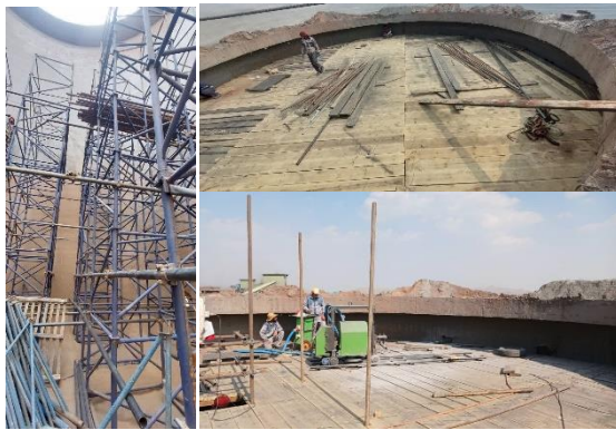
Figure 8. From the right, in order, scaffolding is implemented inside the silos to create a platform for the placement of concrete cutting machines, Chinese planks are placed on the scaffolding to place concrete cutting equipment, and concrete cutting equipment is placed.
