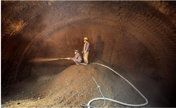
Figure 4. Dry mix Shotcrete
