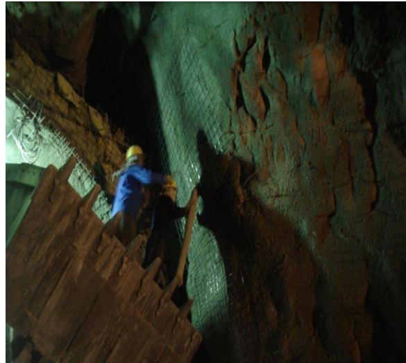
Fig. 2. Implementation the Initial orthogonal mesh reinforcements
