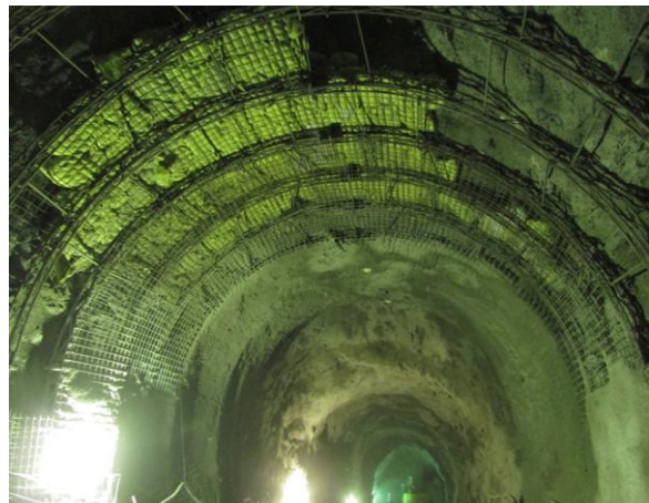
Fig. 3. Implementation the profile frame
