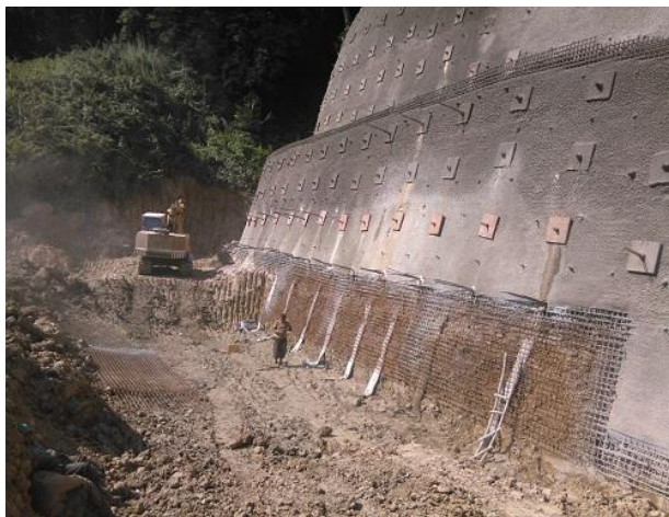
Fig.1 stabilization of earthen wall by nailing method
