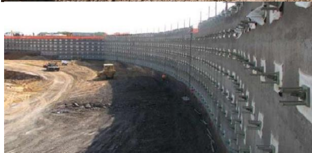
Fig.2 stabilization by a combination of nailing and anchorage method
