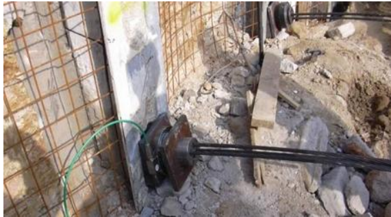
Fig 12. The steel strands installed and the grouting is done and the earthen wall should be cover by spraying concrete.
